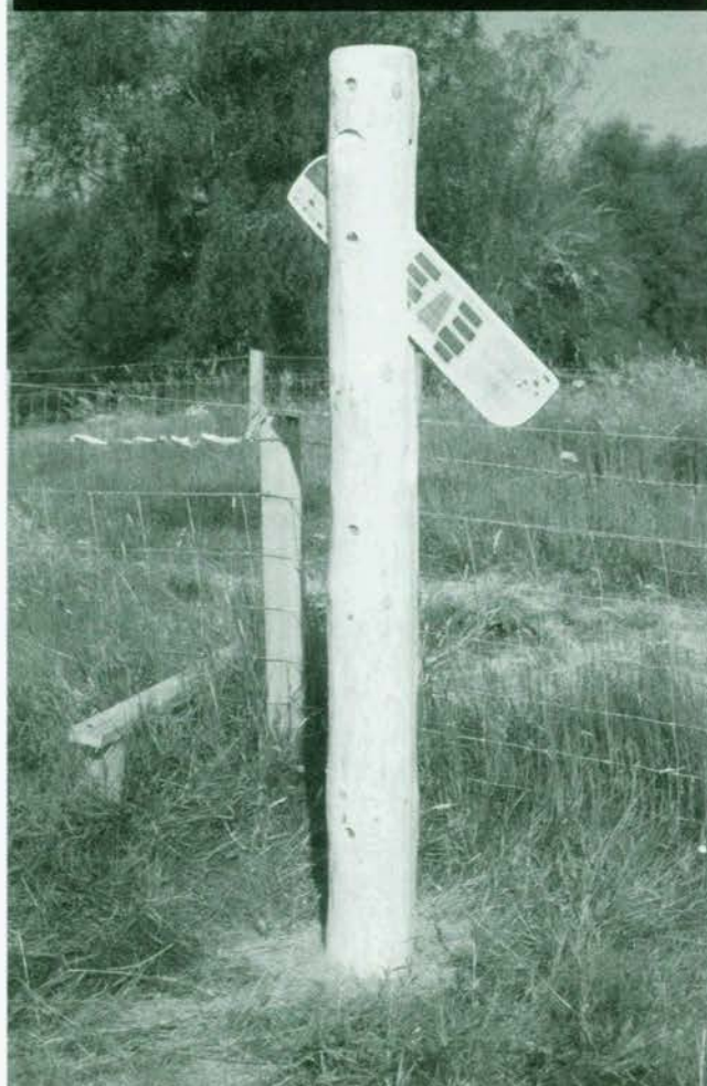
An enterprise, non-invasive 'signalpost' sign. The 'panel' - the signal arm-rests inside the body of the post, protected from nasty UV rays and weather!
