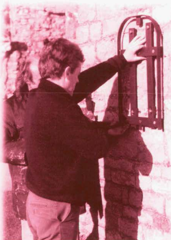
Erecting a new panel: levelling the frame on the wall. The panel is then slid up into the frame
